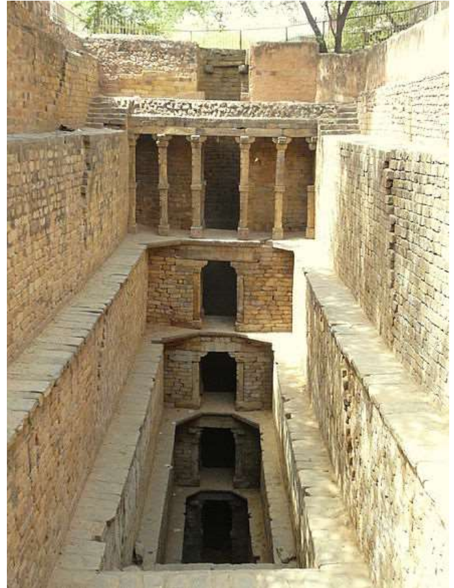
(a). Gandhak Ki Baoli of India in dry condition ( https://en.wikipedia.org/wiki/Baolis_of_Mehrauli )
