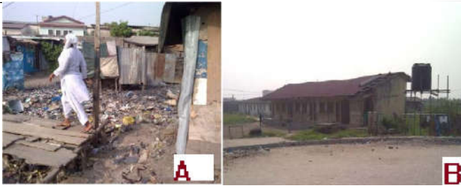
Figure 3. Wooden Platform over Stagnant Water owing to Lack of Drainage (A) and The Government Secondary school in the area (B) Source: Authors' Survey
