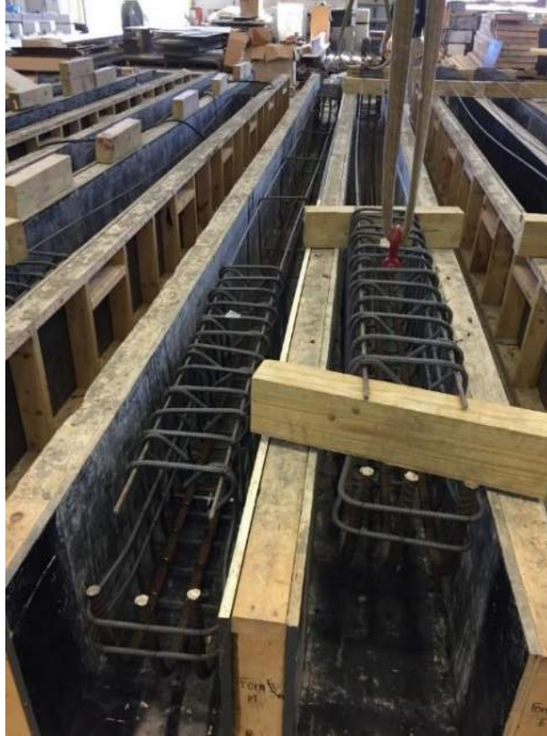
Figure 4.18: Beam Shear Region and Cage Lifting
