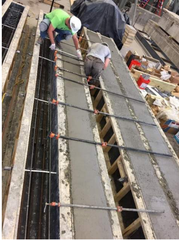
Figure 4.23: Series VI Form Bracing
