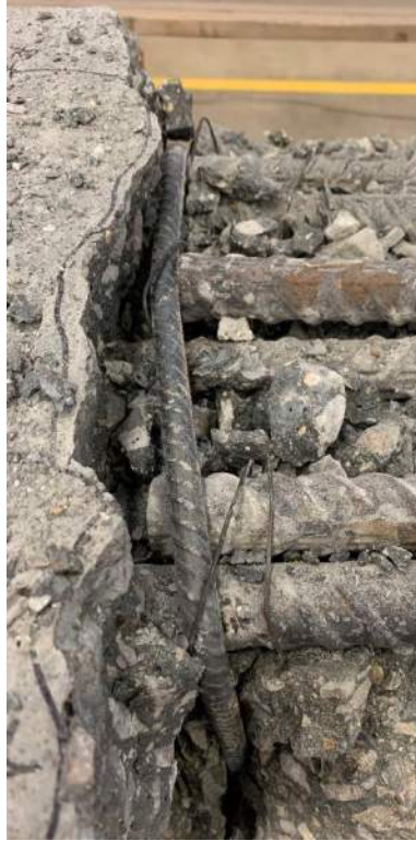
a) South End of Splice
