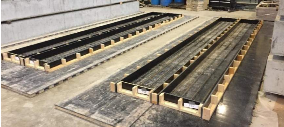
Figure 3.11: Series V Completed Formwork
