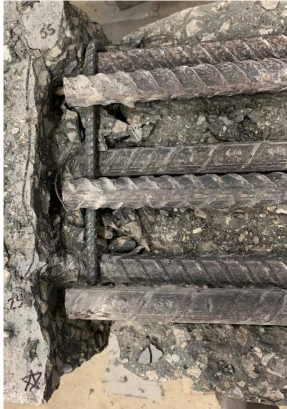
Figure 4.56: Bar Slip on Specimen C3/60/2-40-10-25
