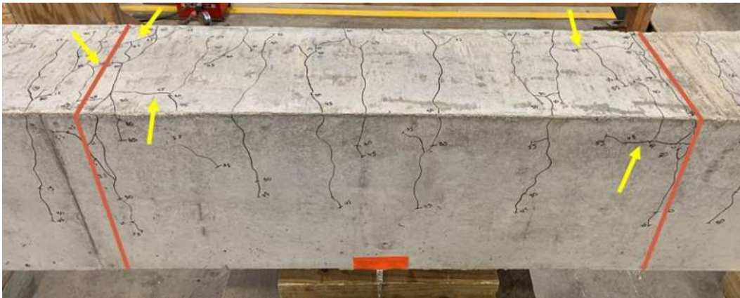
Figure 4.51: Longitudinal and Branch Cracking Before Flexural Failure (C3/60-50-5-200)
