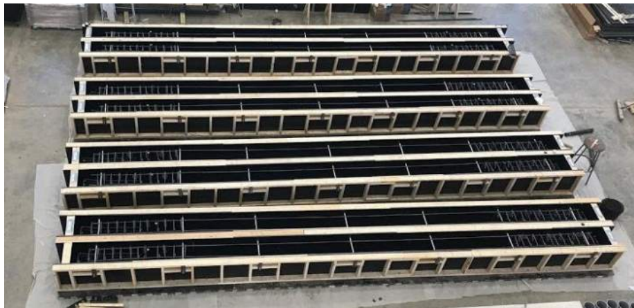
Figure 2.16: Completed Formwork
