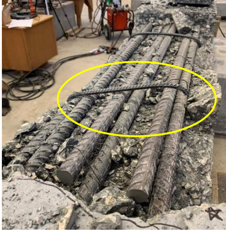
Figure 4.58: Ruptured Stirrup on Specimen C3/60/2-40-10-50
