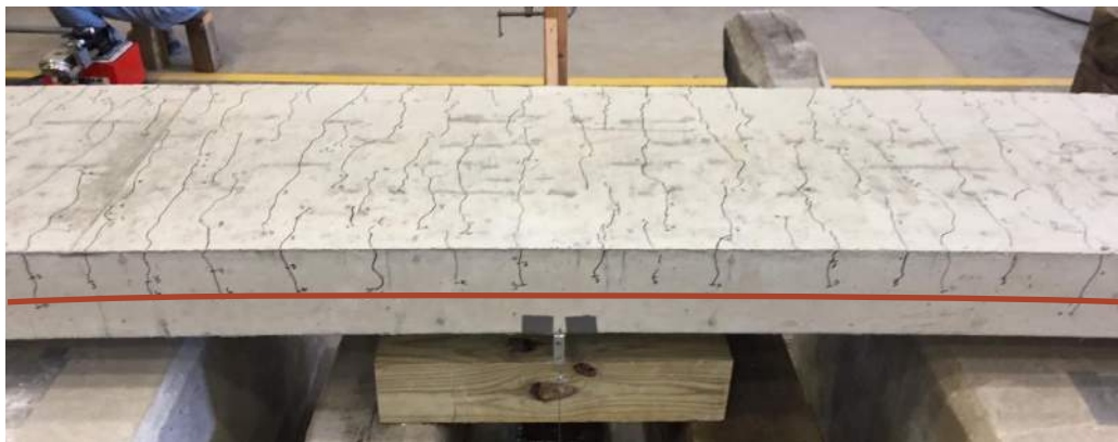
Figure 3.41: Side Crack Propagation (S-100-5)
