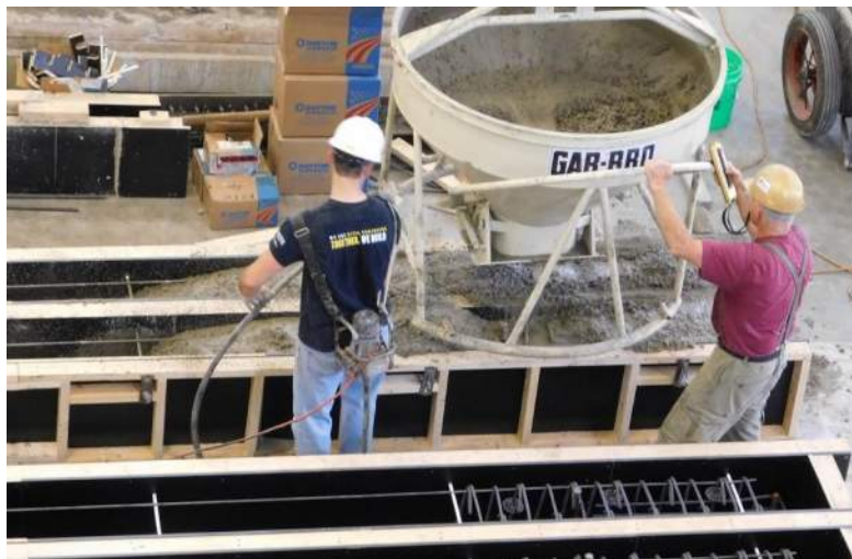
Figure 2.19: Casting Procedure for Specimens
