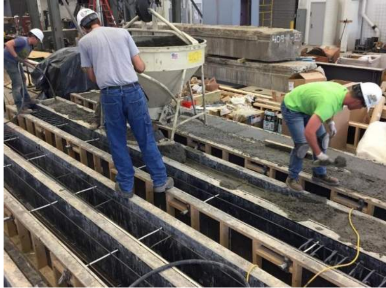
b) Casting In Progress
