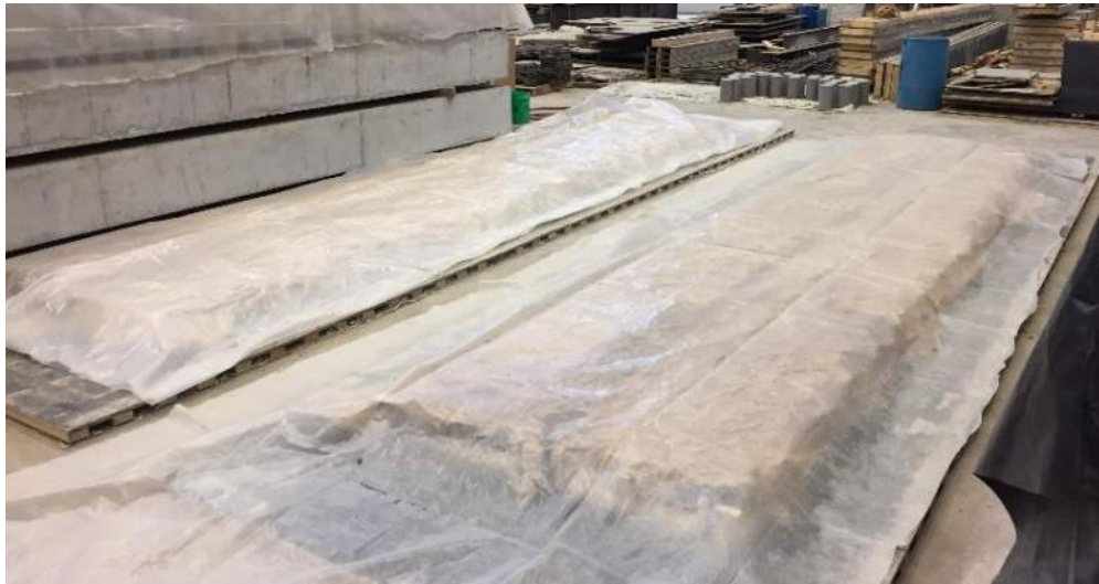
Figure 3.19: Series V Moist Curing
