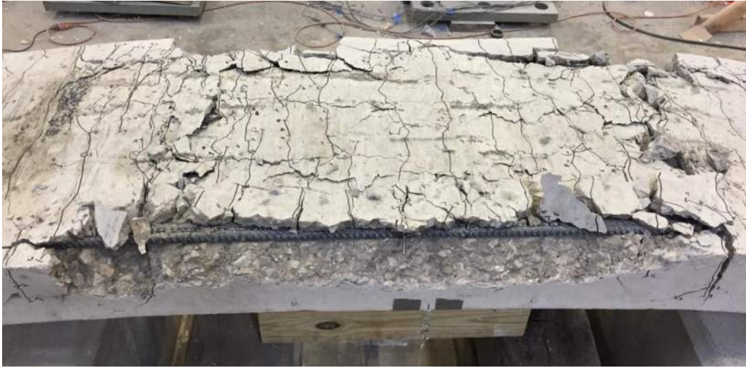
Figure 3.48: S-60-5 Final Failure
