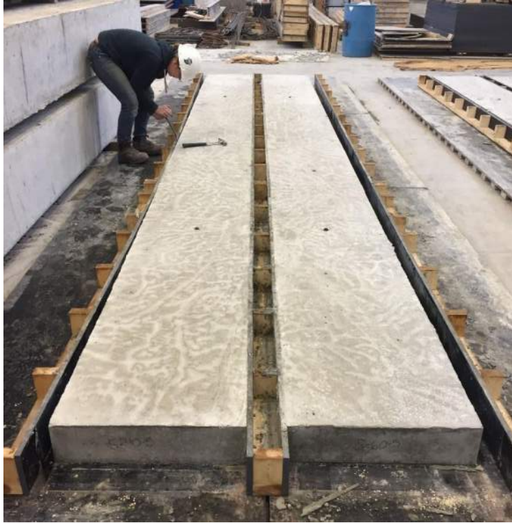
Figure 3.20: Series V Side Form Removal
