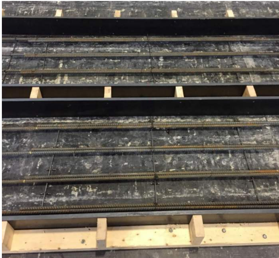
Figure 3.13: Slab Construction – Splice Region
