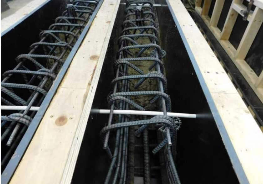
Figure 2.17: Reinforcing Cages Inside Forms
