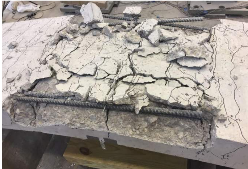
Figure 3.45: S-40-5 Face- and Side-Splitting Failure
