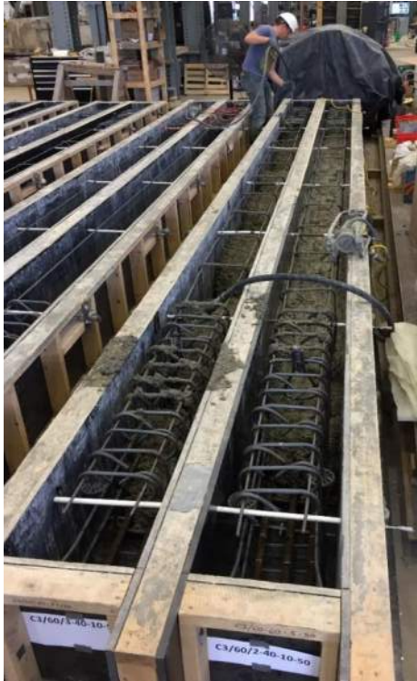
a) Half-Beam Casting
