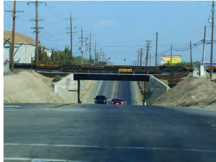
Figure 1.18 The railroad bridge and the "dip" are unattractive features on the east entrance to town.
