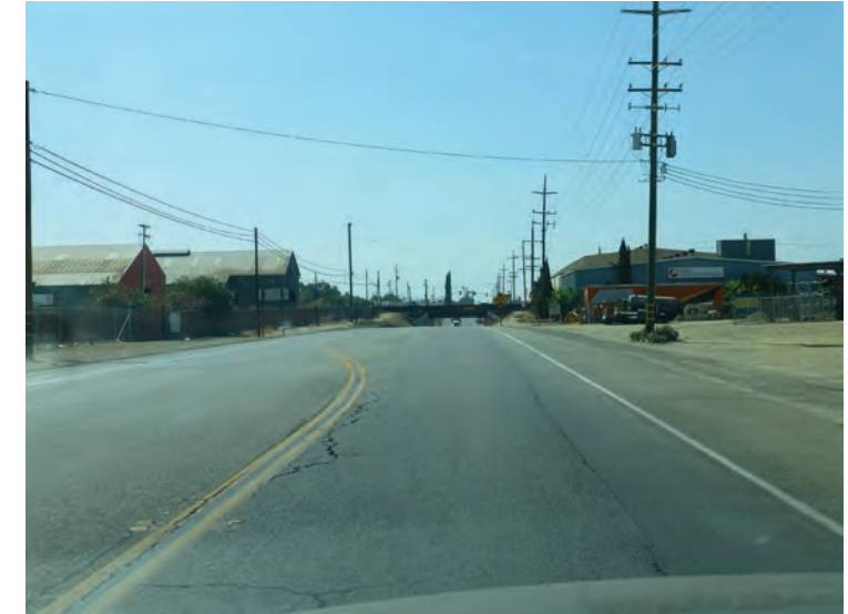
Figure 1.20 The east entrance to town, with the "dip" and the rail bridge coming up, is marked by poorly maintained underutilized industrial lots and buildings.
