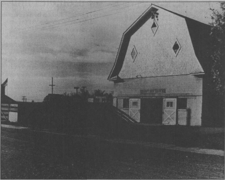
THE USU ART BARN, photographed here in the 1940s, was not moved in the '50s when much of the campus was under reconstruction. It was deemed 'too stationary and sentimental to be transported.' /Special Collections and Archives photo
