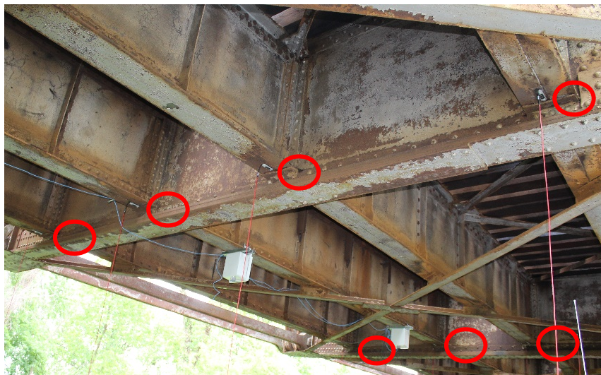
Fig. 24 Installed strain sensors (circled).
