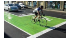
Class II bicycle lanes will be provided, and the option of bike boxes and green painted pavement is available to increase safety and awareness of bicyclists on the road.
