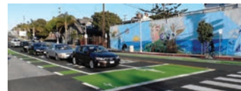
Example of the bike box placed in front of the vehicles at an intersection
