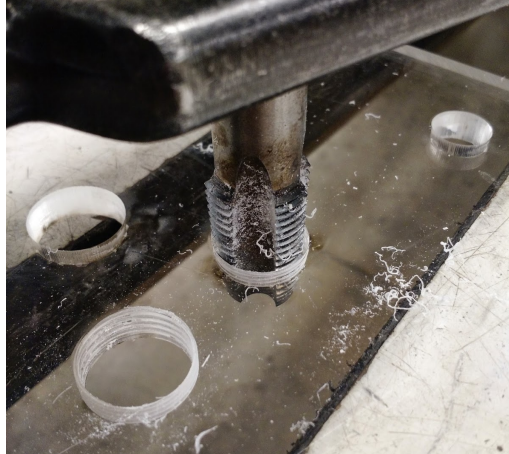
Figure 15. Thru hull connector holes being tapped.
