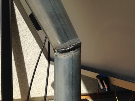
Figure 9 Photo of Modified Metal Pole
