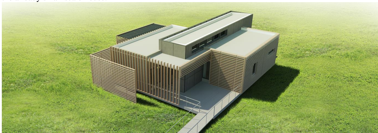
Figure 10. View of the wooden envelope with alternating screen direction to effectively cut down on sunlight.
