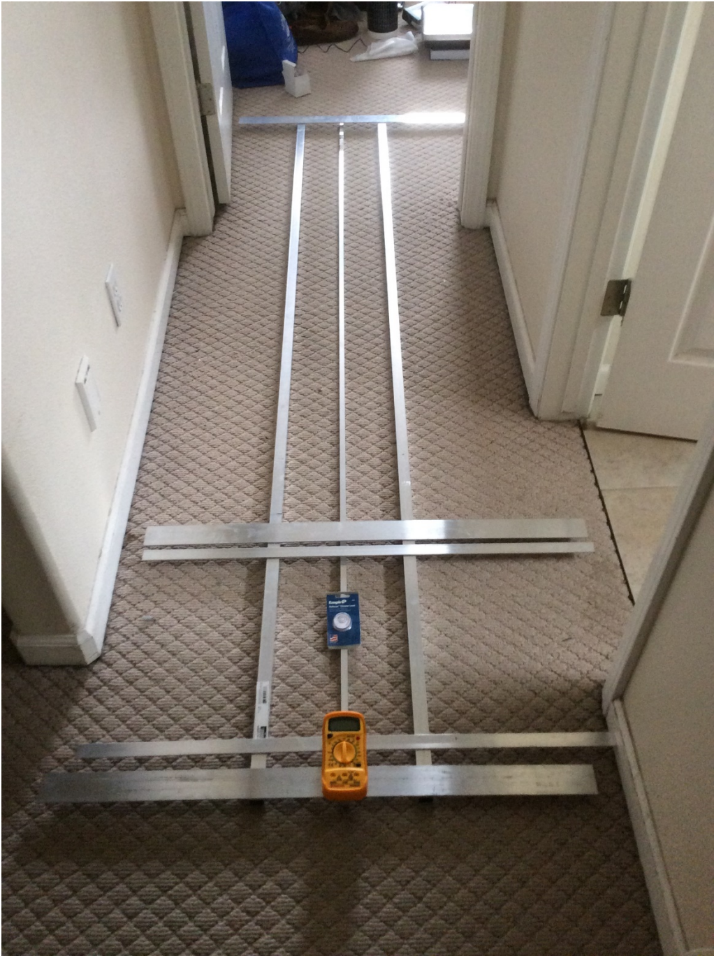
Planning and laying out the Paso Panel Design 5/21/14
