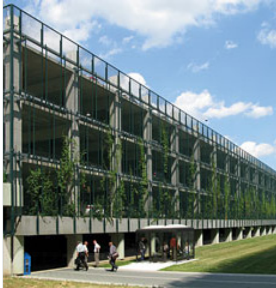
Figure 4.12: Example of parking garage shielding using landscaping that can make such structures more publicly appealing
