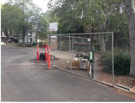
Figure 81: Ugly ongoing construction site
