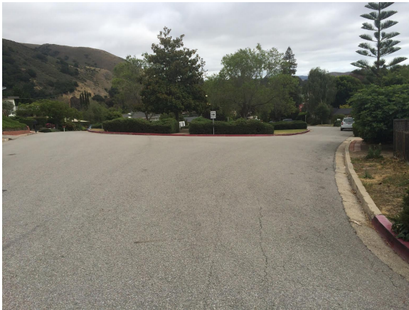
Figure 13: Awkward intersection at the top of Buena Vista Park
