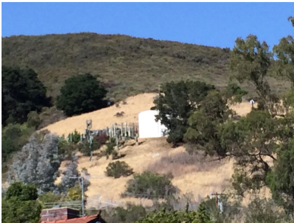
Figure 17: Water storage tank viewshed from Slack Street
