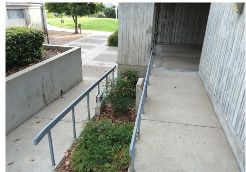
Figure 52: Safe pedestrian ramp
