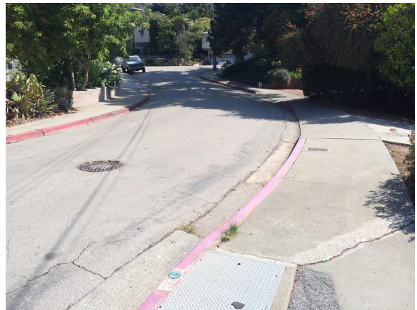
Figure 10: Sidewalks on San Miguel Street
