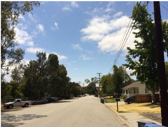
Figure 45: No streetlights on Loomis Street
