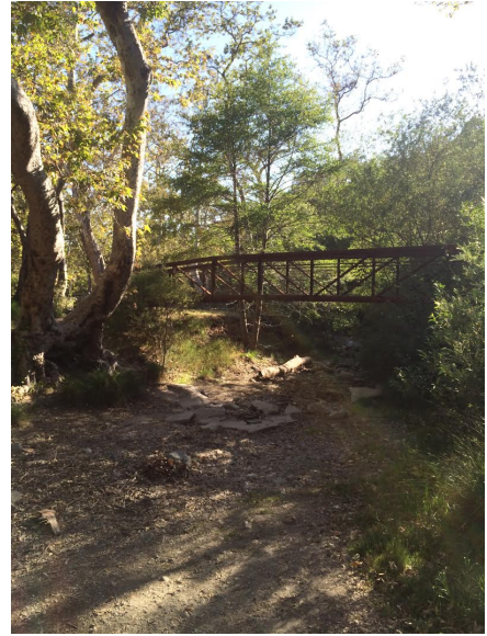
Figure 42: Cuesta Park Bridge
