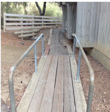
Figure 83: Bridge that is not bike friendly
