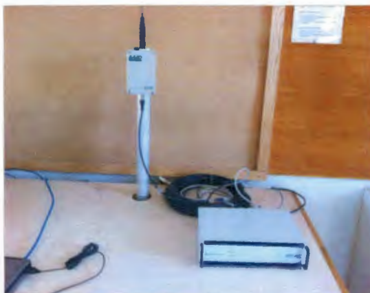
Figure 20: A850 Gateway at the Water Resources Facility
