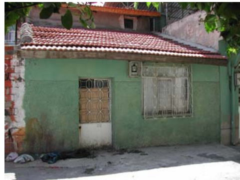
Figure 3.74. Single storey refugee house (387th Street No.14)
