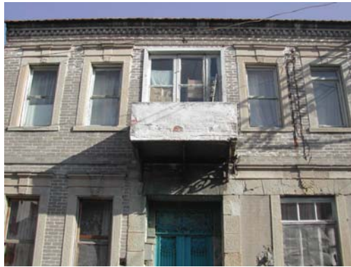
Figure 3.64. Cumba converted into balcony (384th Street No. 65)
