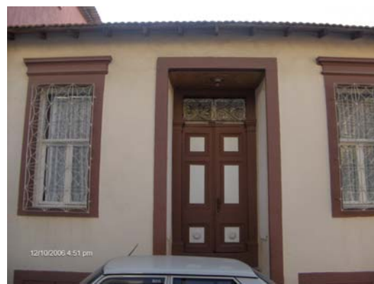
Figure 3.29. Two winged, wooden door (377 Street Street No. 2) The door the inserted into a slightly deep niche without a vault. There is a fixed rectangular window over the door.
