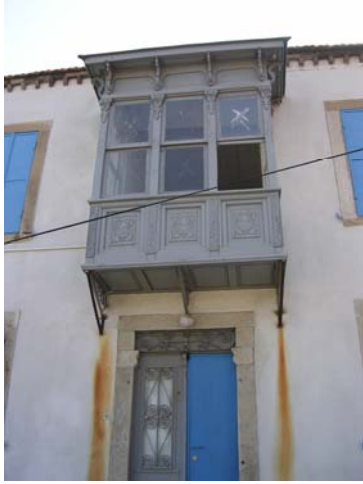
Figure 3.53. Cumba is middle of the façade 403rd Street No. 30
