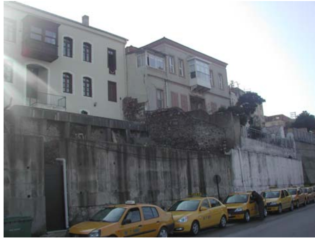
Figure 4.7 View of buildings at 404 Street No. 19 - 21 from Halil Rifat Paşa Street
