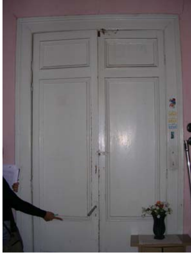
Figure 3.11. First floor, the wooden closet in the hall (400th Street No. 13)
