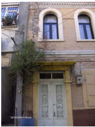
Figure 3.57. Plain cornice between upper and lower floors (377th Street No. 8)
