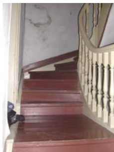
Figure 3.18. U-type wooden stairs, Halil Rifat Paşa Street No. 74
