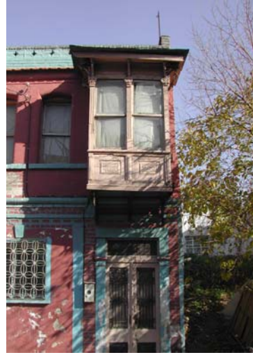
Figure 3.49. Wooden cumba has two vertical section and three horizontal section (384th Street No. 59)
