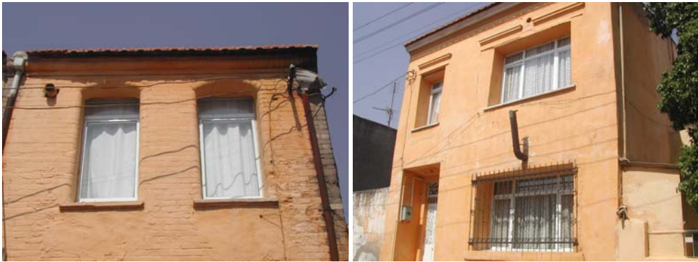
Figure 3.66. Alterations in window dimensions and materials
