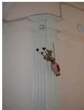
Figure 3.14. Ground floor, on the wall corner, 384 Street
