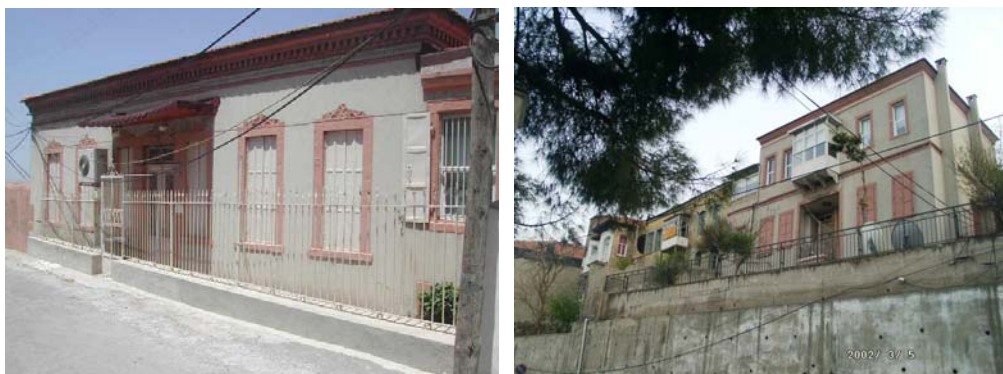
Figure 3.68. View from Halil Rıfat Paşa Street of the double floor façade of the building which seems to have just one single floor when looked at from 404th Street
