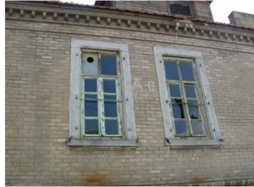
Figure 3.56. Perforated eave cornice (397th Street No. 29)
