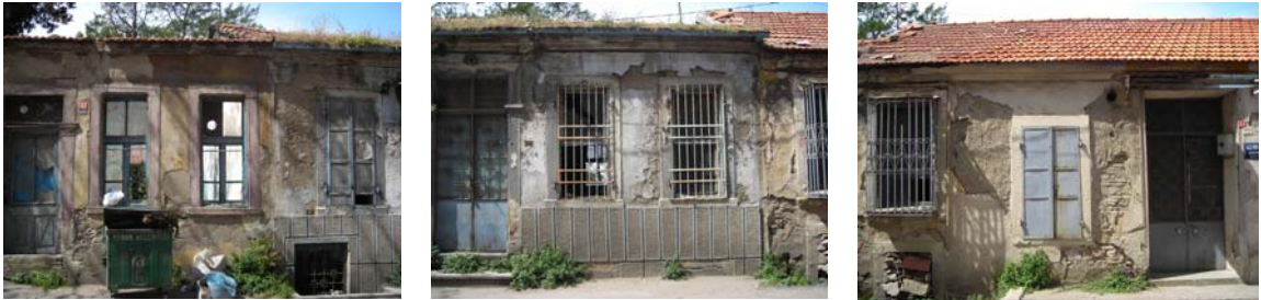
Figure 4.13 Ruined buildings at Halil Rifat Paşa Street Nos. 44 – 46 – 48
