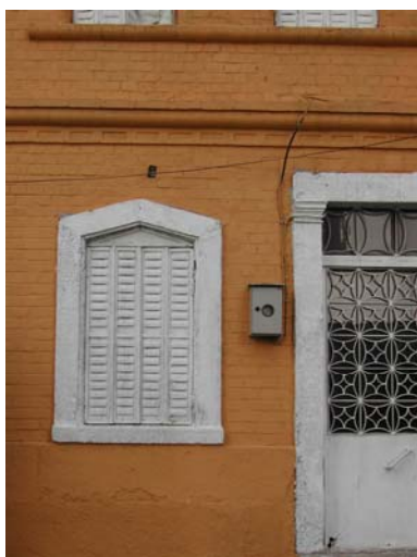
Figure 3.43. Window with iron shutter and its above a triangle jamb (Halil Rıfat Paşa Street No. 83)
