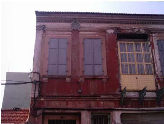
Figure 3.59. In this building, the eave cornice is constructed in a perforated form under the plain finishing. The vertical corner finishing in this building is in a column form and it is connected to the floor finishing by preserving it along upper floor's height in stead of eliminating it on the second floor. (384th Street No. 62)
