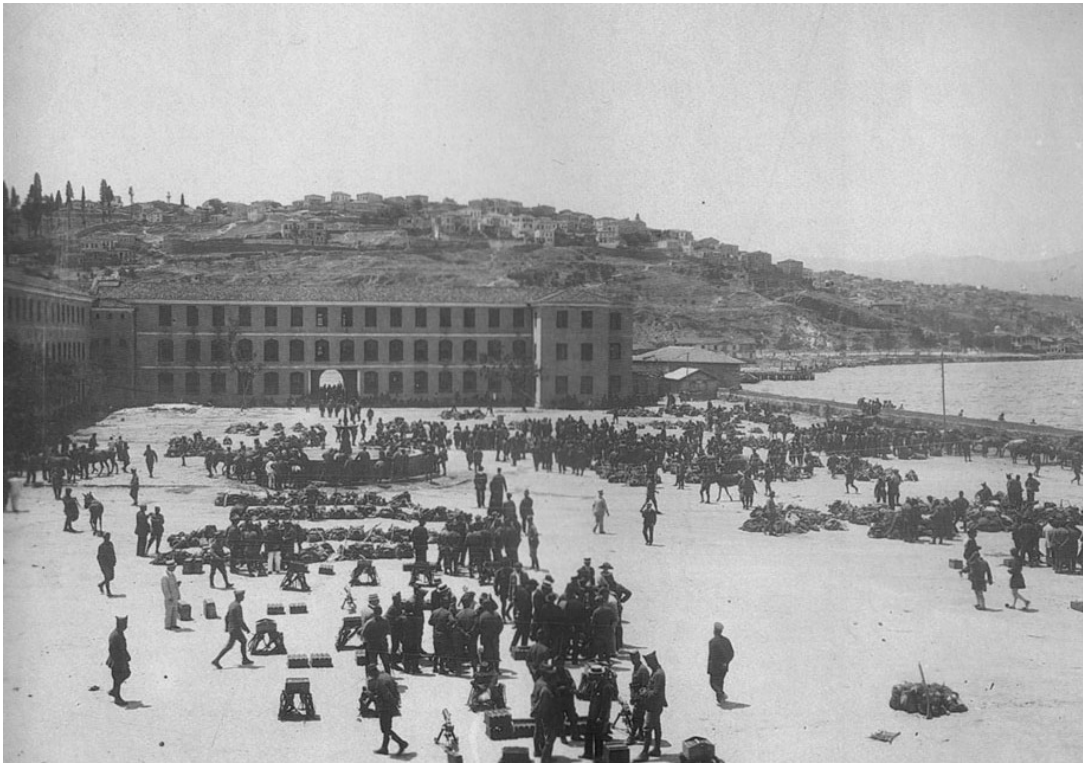
Figure 2.15 A view to Değirmendağı from Sarıkışla (Source: İzmir City Archives)
