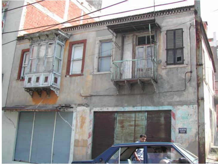
Figure 3.65. Cumba converted into balcony (Halil Rifat Paşa Street No. 60-62)
