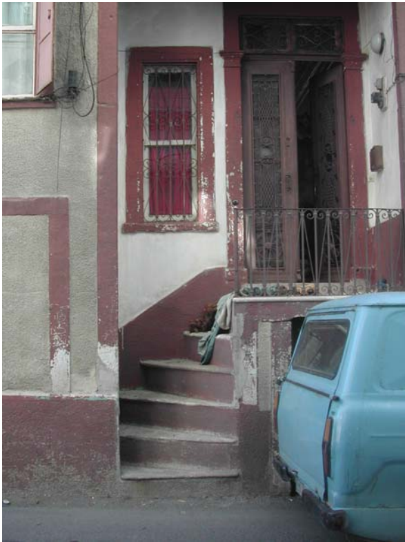
Figure 3.30. Two winged, wooden door (Halil Rifat Paşa Street No. 74) The sub entrance is separate. The niche, covering entire staircase, is pretty deep.
