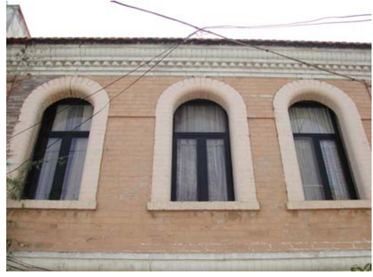
Figure 3.40. Window surrounded by white bricks in a traditional method and corners are softened (377th Street No. 8)
