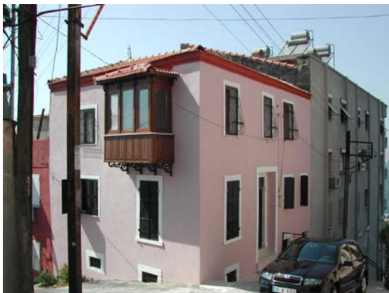
Figure 3.51. Wooden cumba 404th Street No. 6
