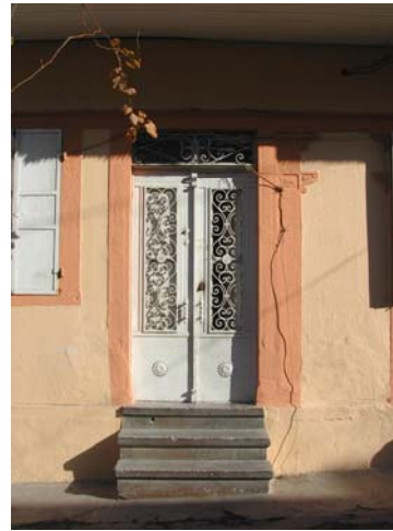
Figure 3.27. Two winged, iron door (384 th Street No. 55)
