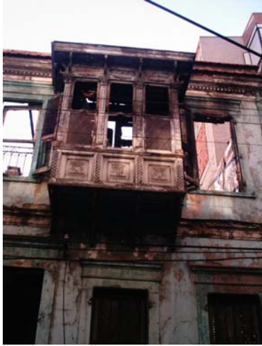
Figure 3.48. Wooden cumba has three vertical section and two horizontal section (Halil Rifat Paşa Street No. 54)
