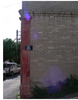
Figure 3.60. Corner column and floor cornice (402nd Street No. 15)
