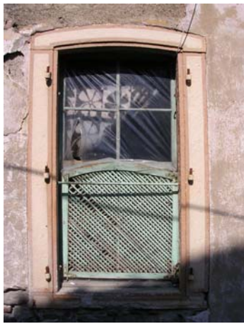
Figure 3.41. Ground floor window with wooden shutter (403rd Street No. 13)
