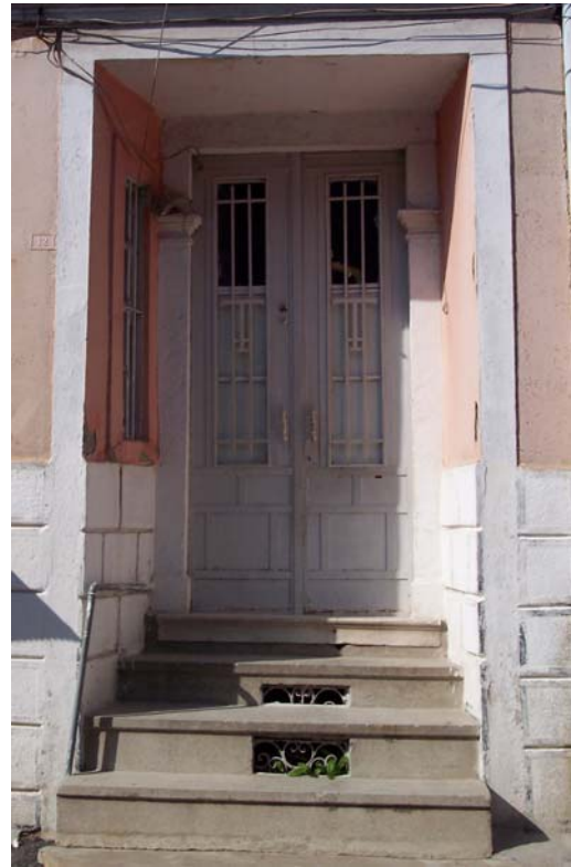
Figure 3.31. Two winged, iron door (400th Street No. 14) The inferior door is massive.
