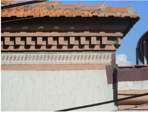
Figure 3.55. Perforated eave cornice (404th Street No. 19)
