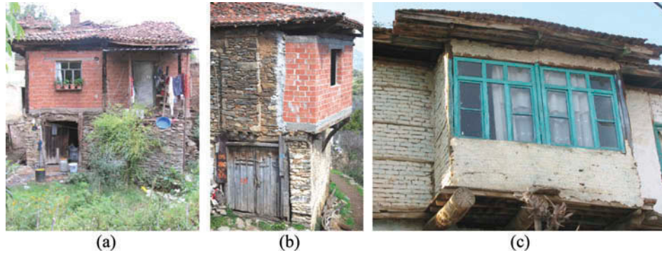
FIG. 26. Spatial changes with: (a–b) RC slab and hollow bricks walls (Beydağ-Alakeçili), and (c) window enlargement of a bay window in hımış frame with brick infill (Kiraz-Karaburç).
