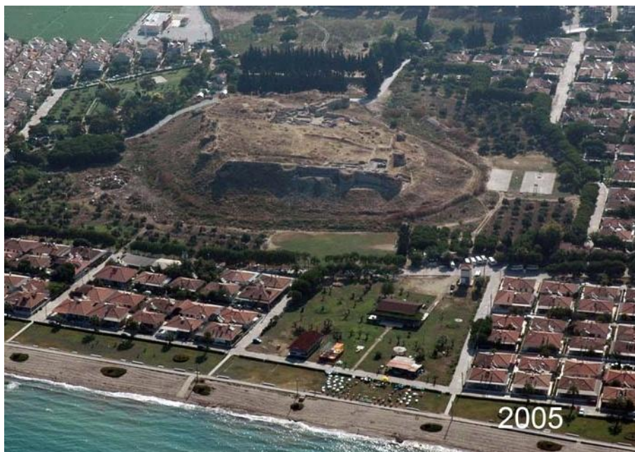
Figure 17. Aerial photograph of Kadikalesi Mound in 2005 (Source: The archives of Anaia Excavation 2010).
