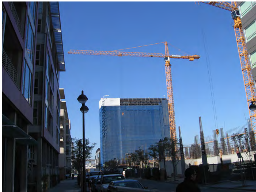
Figure 3.12 Construction Activity in Mission Bay North
