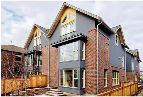
Figure 5.4. TA multi-unit complex in the Boulders, in Seattle, Washington. The complex, like the residential structures in Figure 5.3, were the inspiration for the apartment structure in Alternative 2.
