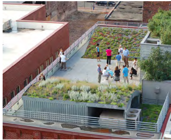
Figure 5.9. Useable roof top
