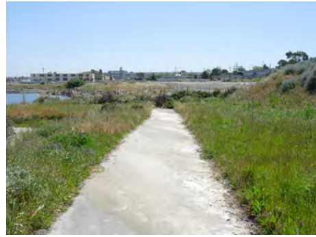
Figure 2.5 Bay Trail - Abrupt End at Site Boundary
