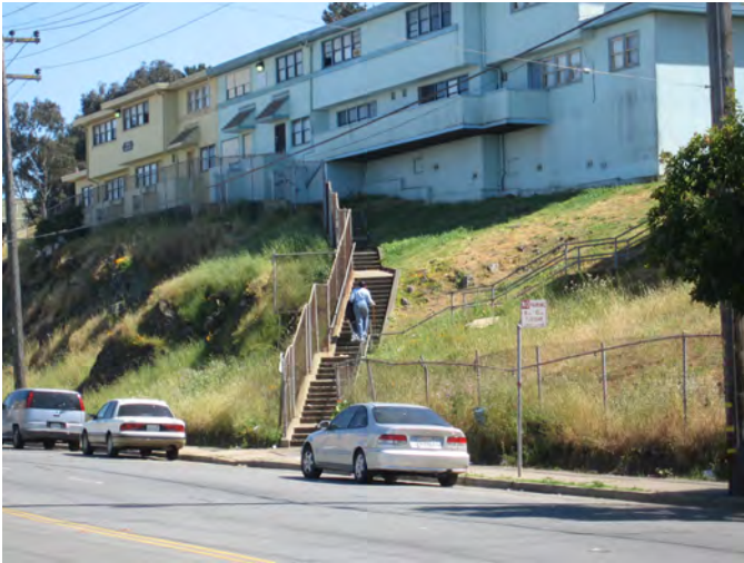
Figure 1-6. Public housing along Innes Avenue.
