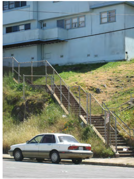
Figure 3.16. Pedestrian Stairway Connecting to Innes Ave.
