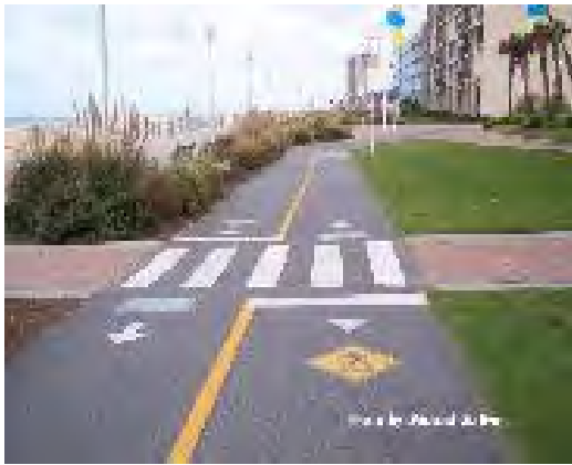
Figure 5.11. Bike and pedestrian path with differentiated pavers to delineate direction and transportation type.
