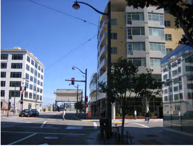
Figure 3.9 Mission Bay North Showing Street Level Retail and Mixed Use
