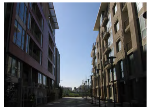
Figure 3.23 Mission Bay North Housing Open Walkway Between Buildings
