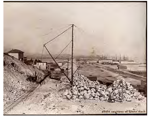
Figure 3.2 Kentucky Street (now 3rd Street) grading work circa 1870 Photo courtesy of Glenn Koch
