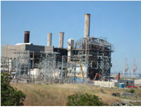
Figure 3.4. Old PG&E Power Plant
