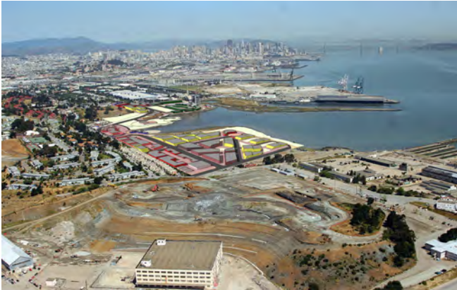
Figure 4-2. Aerial view of India Basin Shoreline from Shipyard.
