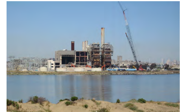
Figure 2-5. PG&E switch station/transformer.
