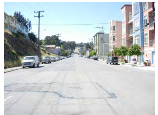
Figure 2.20 Innes Avenue Looking South
