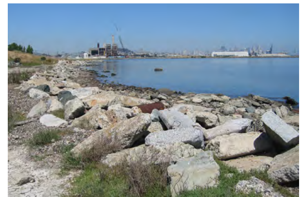
Figure 2-17. Rip-rap to stabilize shoreline and prevent erosion.
