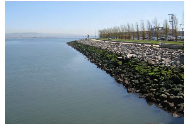
Figure 3-6. Steep slope protection, LEED credit 8.
