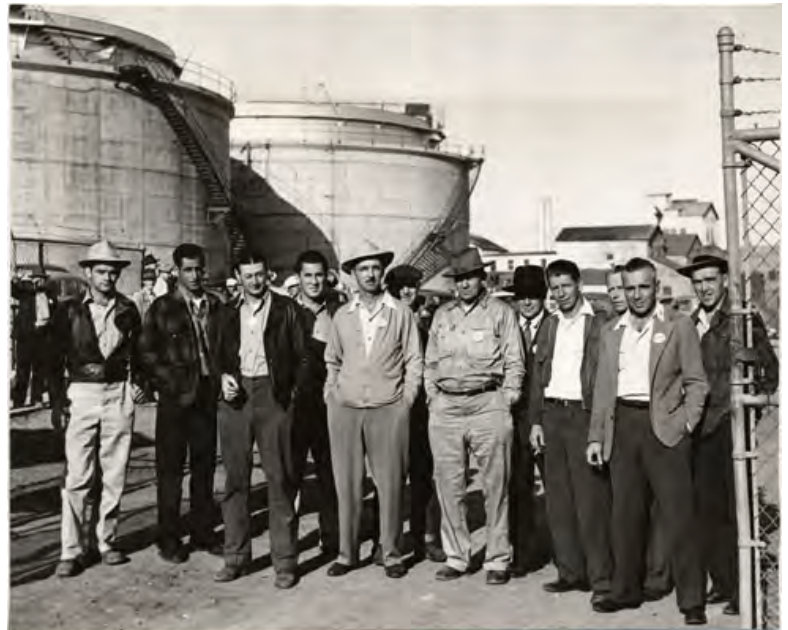
Figure 2.17 Entrance to Pacific Gas & Electric Company Steam Plant Located at the Corner of Jennings Street and Evans Avenue, 1948 Photo Courtesy of San Francisco Public Library
