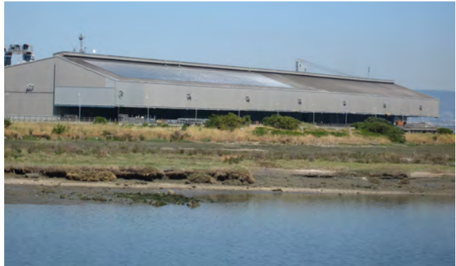
Figure 2-2. Recycling facility across from India Basin Shoreline.
