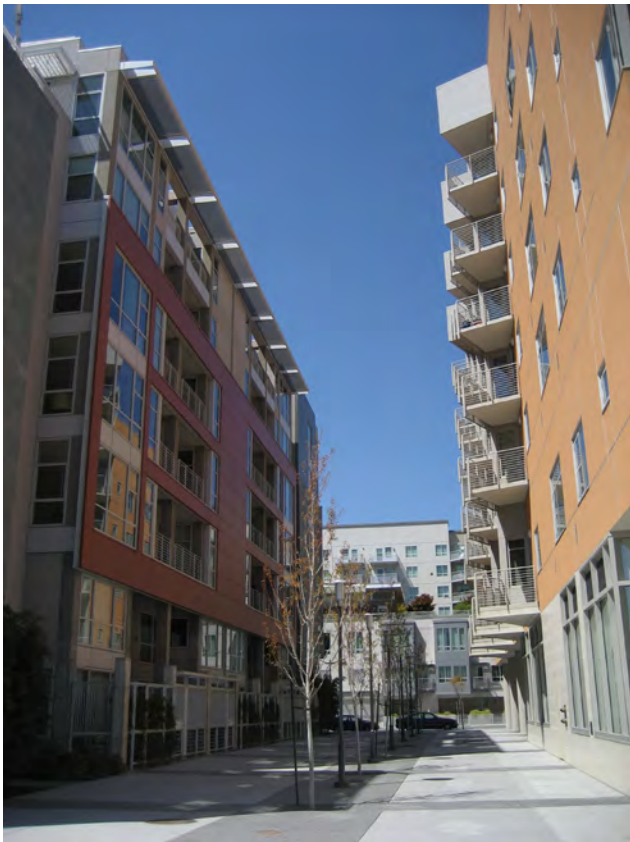
Figure 2.7. A pedestrian corridor between two residential buildings. The buildings are close, creating a sense of privacy for pedestrians.
