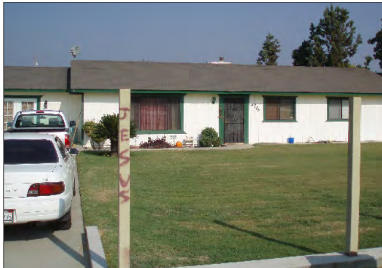
Image X: Average parcels consisted of structures that appeared to be in a fair condition, possibly needing some maintenance, but otherwise structurally sound and completely habitable.
