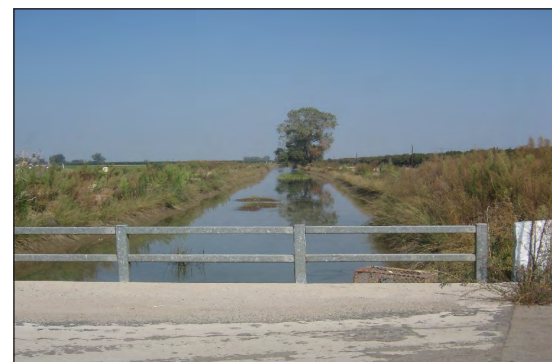
Image X: Canal being used to prevent flooding of community.
