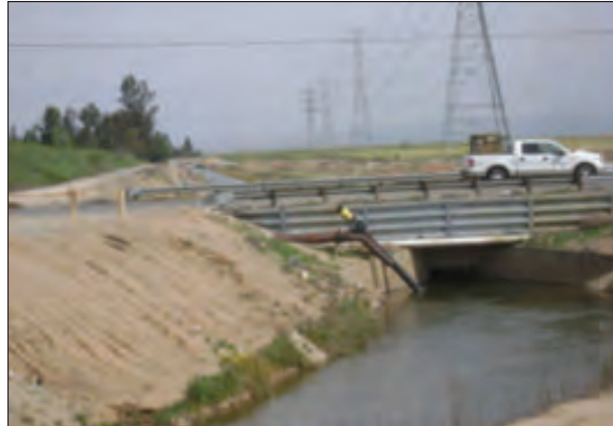
10: At the east access to Madera Ranchos on Avenue 12, the bridge over the canal. There is no indication that one is driving into the community.
