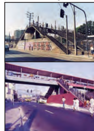
Before and after of pedestrian bridge.
