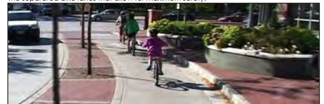
The separated bike lanes that allow for maximum safety.
