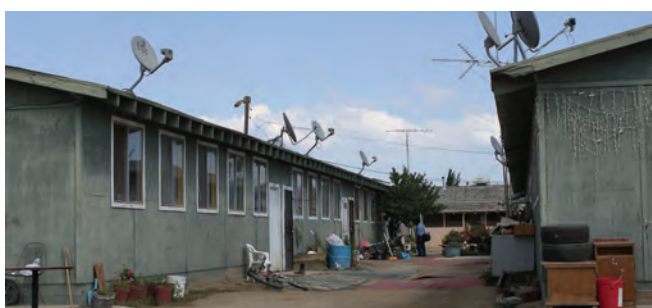
Fig. 3.14: An existing multi family housing.
