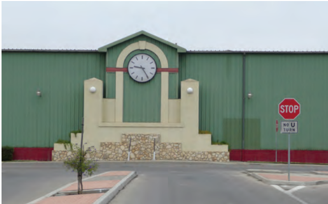
Fig. 3.16: King City depot terminates Broadway.
