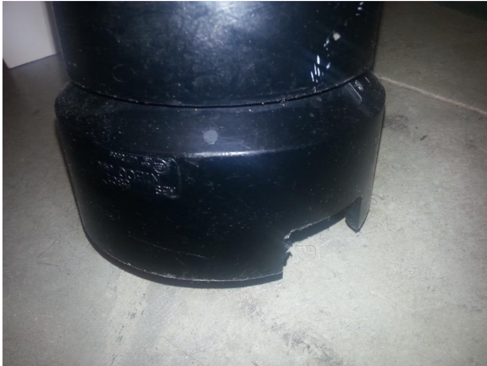
Figure 7. The lower pipe fitting has slots to allow for proper flow regardless of the position in the pit
