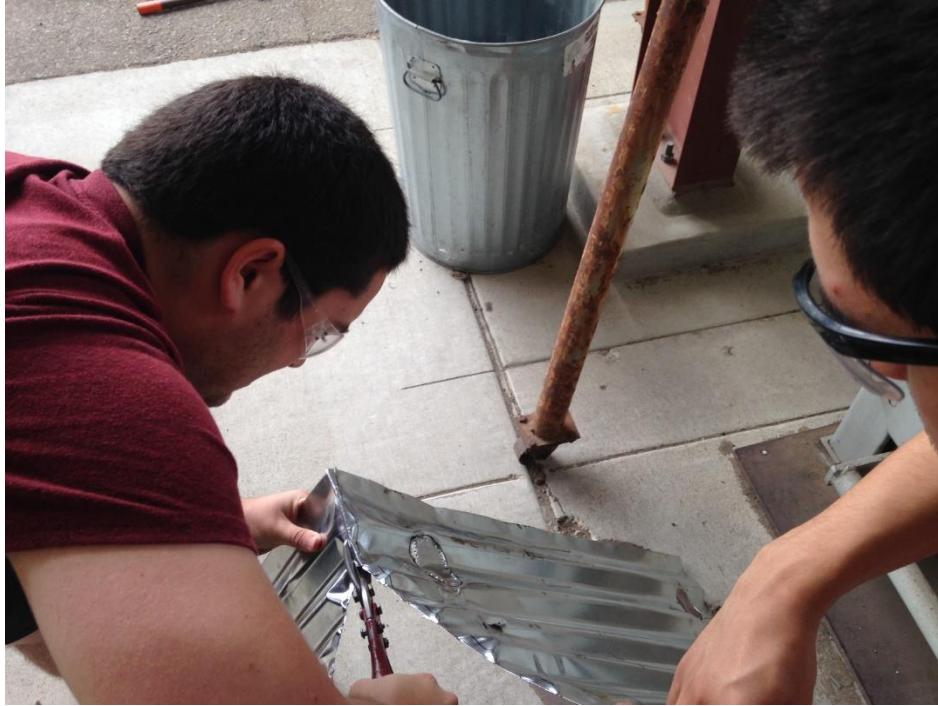
Figure 12. The hole for the water bottle was cut using a circular punch and tabs were formed using a hammer and chisel
