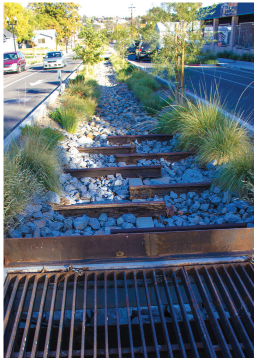
Figure 10: The main detention basin to collect and slow down the flow of stormwater
