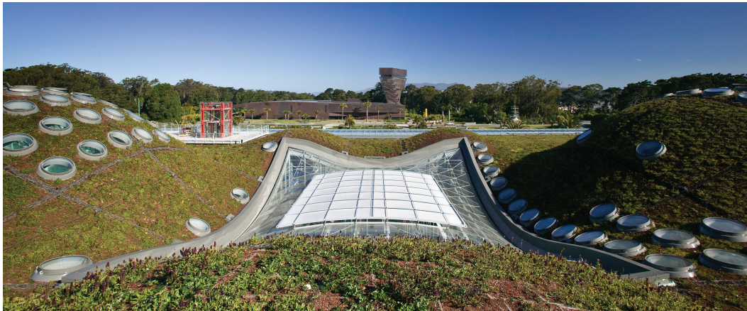
Figure 2: Green roof located on the California Academy of Sciences building
