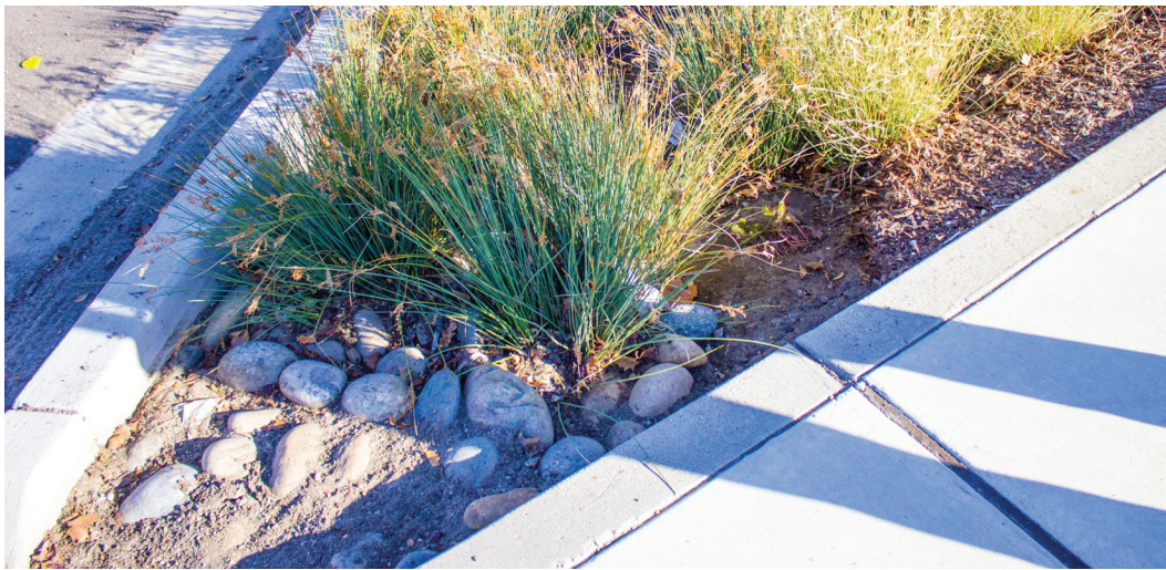
Figure 14: After its first rainstorm, it had already started to collect sand in the planters
