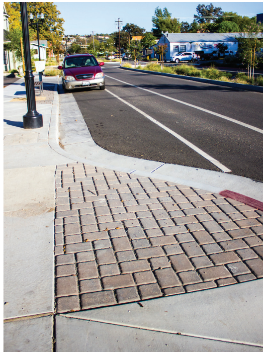
Figure 3 : Permeable paver sidewalk
