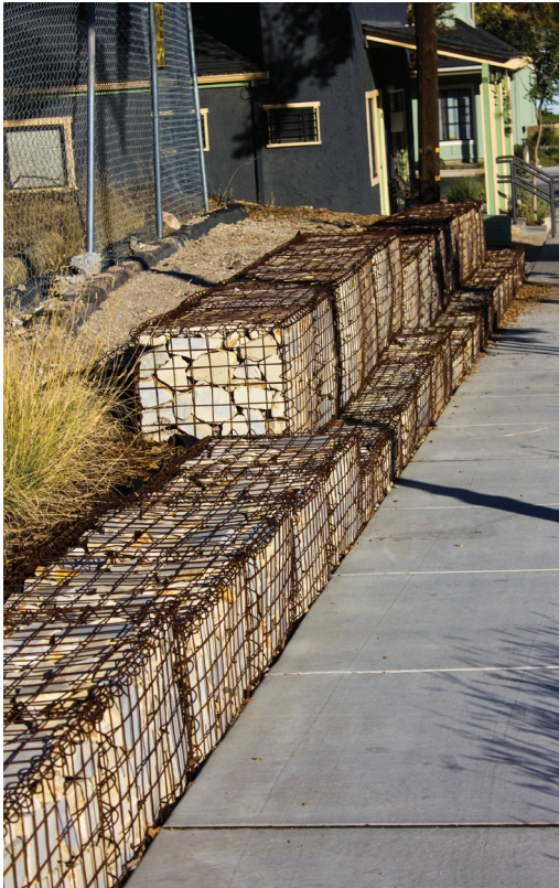
Figure 12: Public benches that also second as a way to reduce the amount of runoff from parcels
