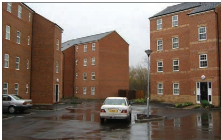
Figure 1: The fashion for neovernacular style can be an excuse for poor quality housing – it is cheaper to provide small windows.
