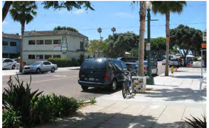
Figure 3-10: Example of attractive and functional sidewalk in Encinitas, CA. Note tile design on planter boxes.
