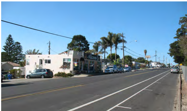
Figure 2-11: View looking west along Shell Beach Road. Note side parking, bike, and traffic lanes.
