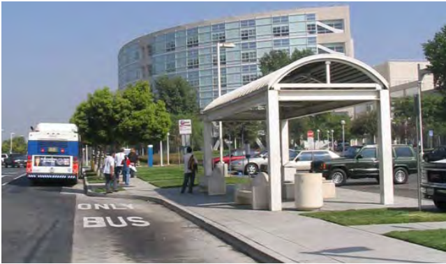
Figure 3-6: Bus turnout with well-established stop.
