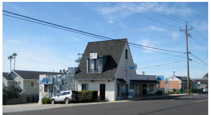
Figure 2-4: Office and commercial buildings along Shell Beach Road
