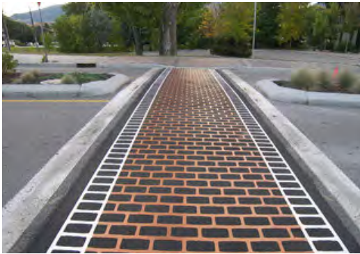
Figure 4-15: Dura-therm asphalt inlay applied to a pedestrian crossing
