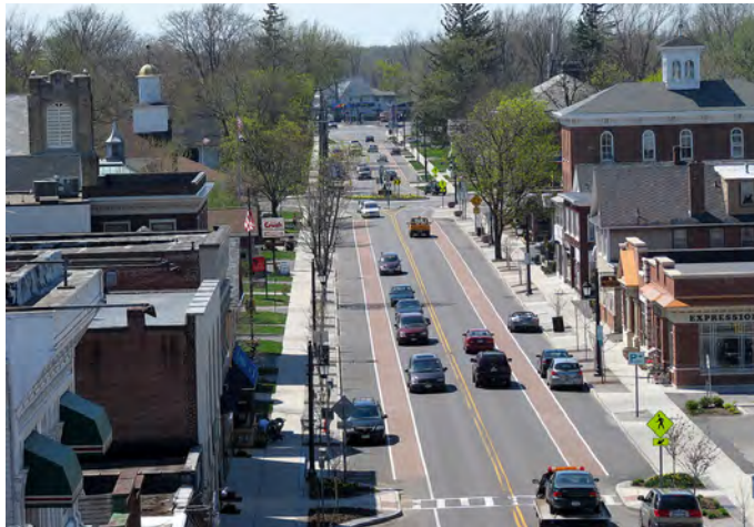
Figure 3-4: Image of an “complete street” showing delineated bike lanes, marking pedestrian paths, and wide sidewalks.
