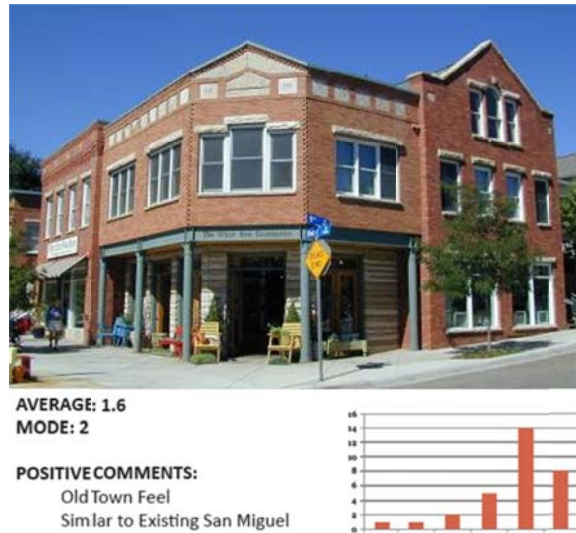
Figure D-4: Mixed-use development with old-town style architectural style and limited height.
