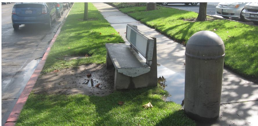
Figure 8: The Cypress at Nicholson bus stop does not have an appropriate landing pad or adequate space on the sidewalk.
