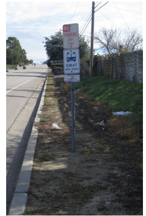
Figure 9: Santa Maria Way at Holly Oak stop with no pedestrian connections.
