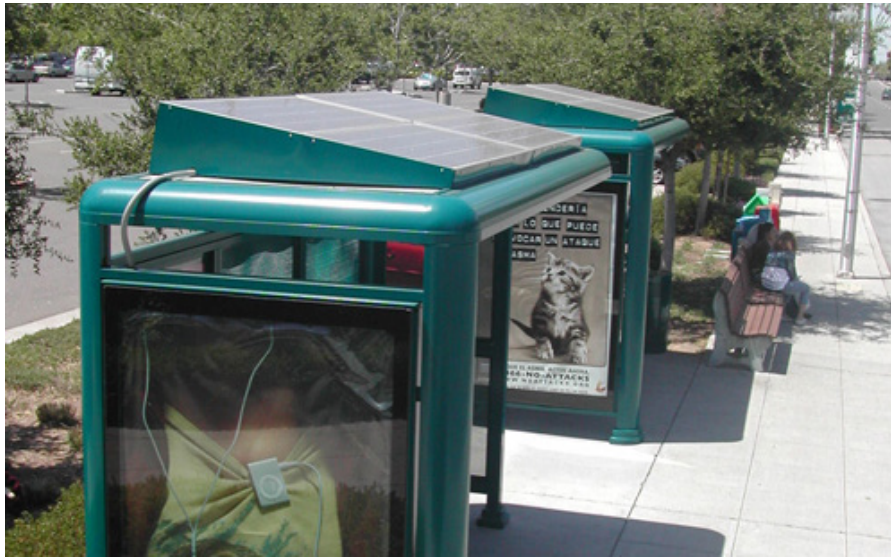
Figure 6: Solar lighting used for evening shelter and advertisement lighting. Source: Apex Lighting
