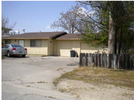
Figure 3.6 Residential Structure on North side of 12 th Street.
