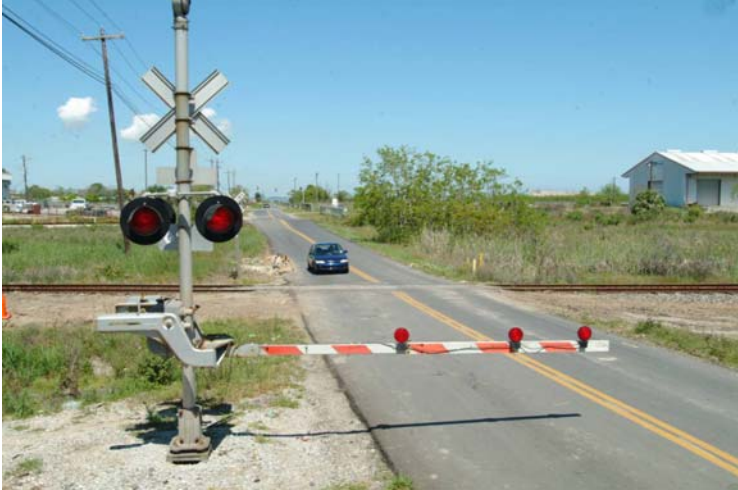
Figure 6.9: Railroad crossing with signals and arms.
