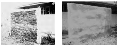
Figure 52: Alternative Adobe Wall Before and After Application of Stucco
