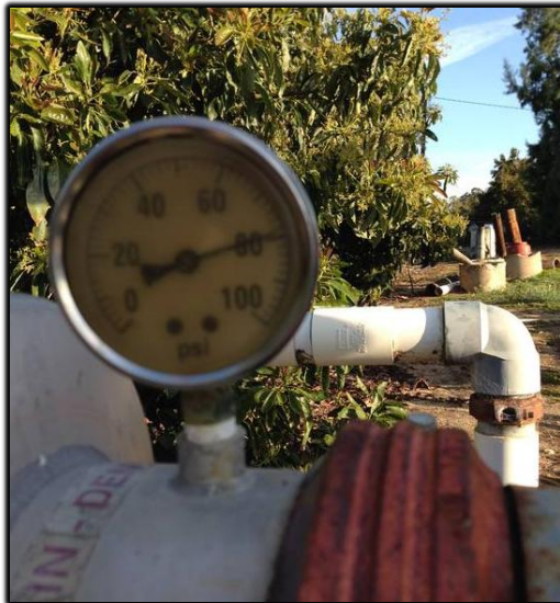
Figure 9. Pressure reading downstream of filter.
