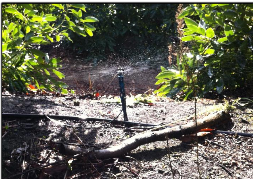
Figure 11. Example of micro-sprinkler in orchard.
