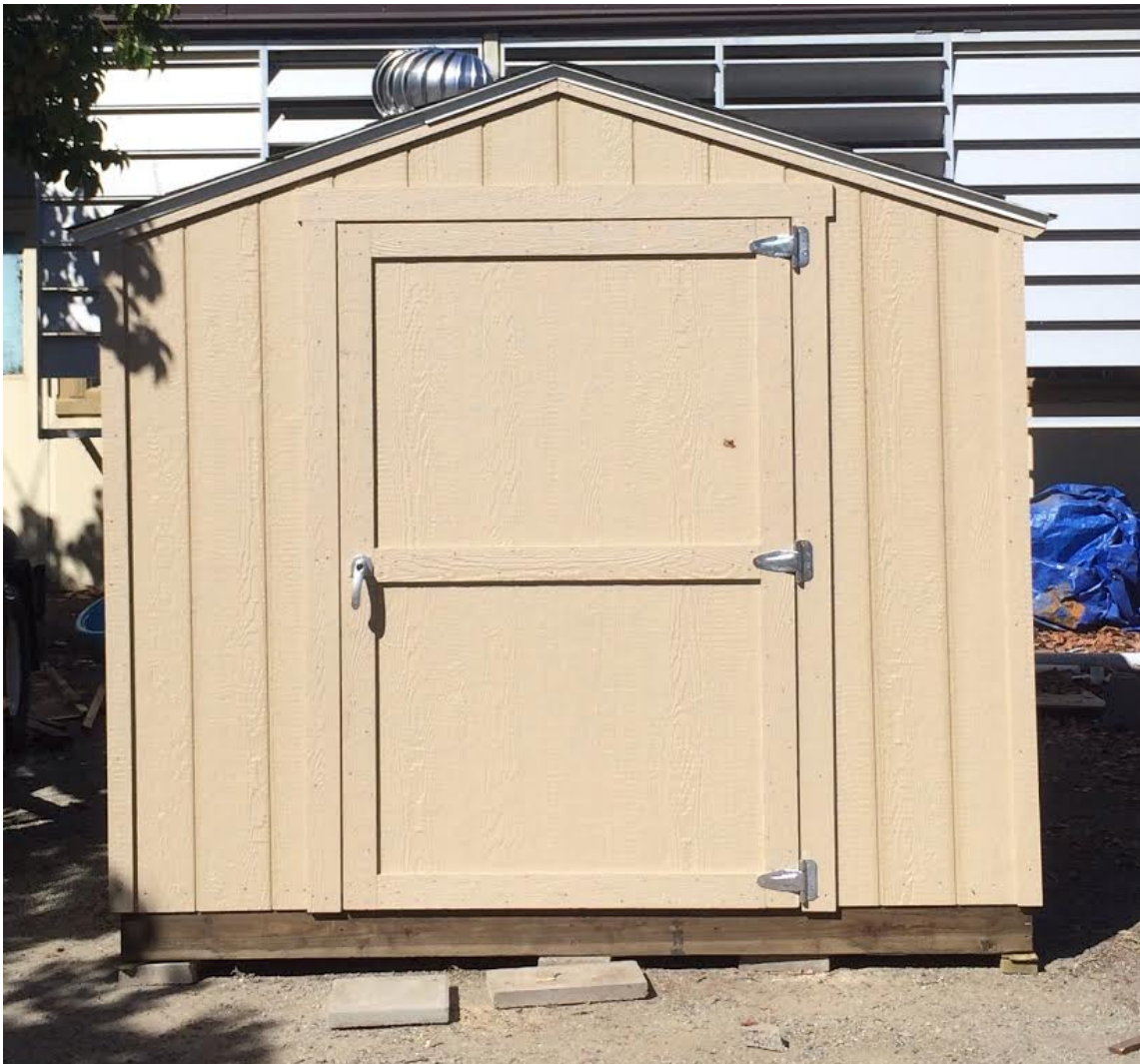
Figure 4-1: DC House (prior to installation of solar panel)
