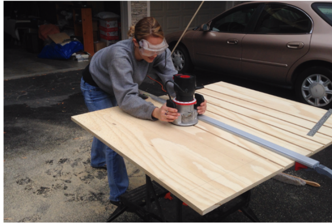
Figure 32: Creating slots for adjustable interior walls.
