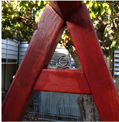
Figure 4-2: Small crossbar supporting the bearing
