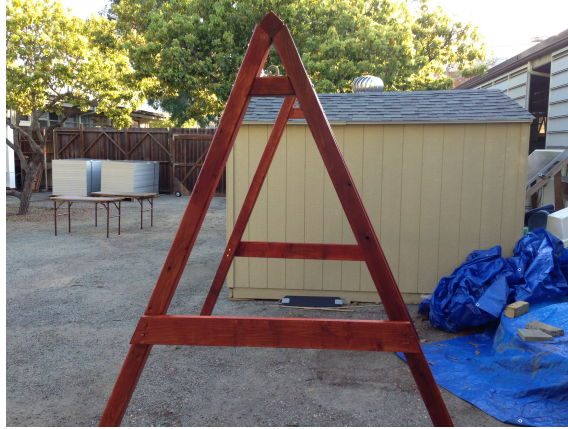
Figure 4-1: Side view of the swing structure with the A frame formation
