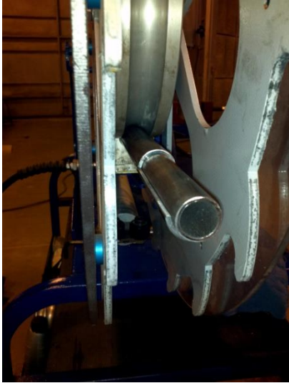
Figure 9.47 - Getting ready to bend the main roll hoop. Both the one inch and 1.25 inch tubes can be seen.
