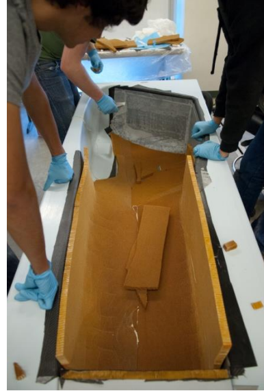
Figure 9.20 - Placing the core in the mold. The white seams are film adhesive used to splice sections of core together.
