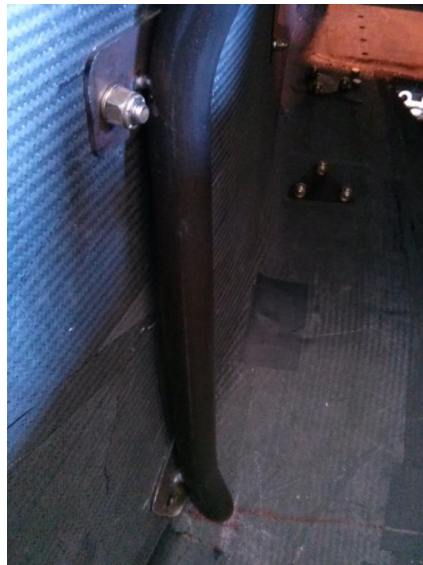
Figure 9.56 - Showing how the front roll hoop attaches to the sides of the monocoque. There is an equally sized plate on the outside of the tub to spread the load out over a larger area.
