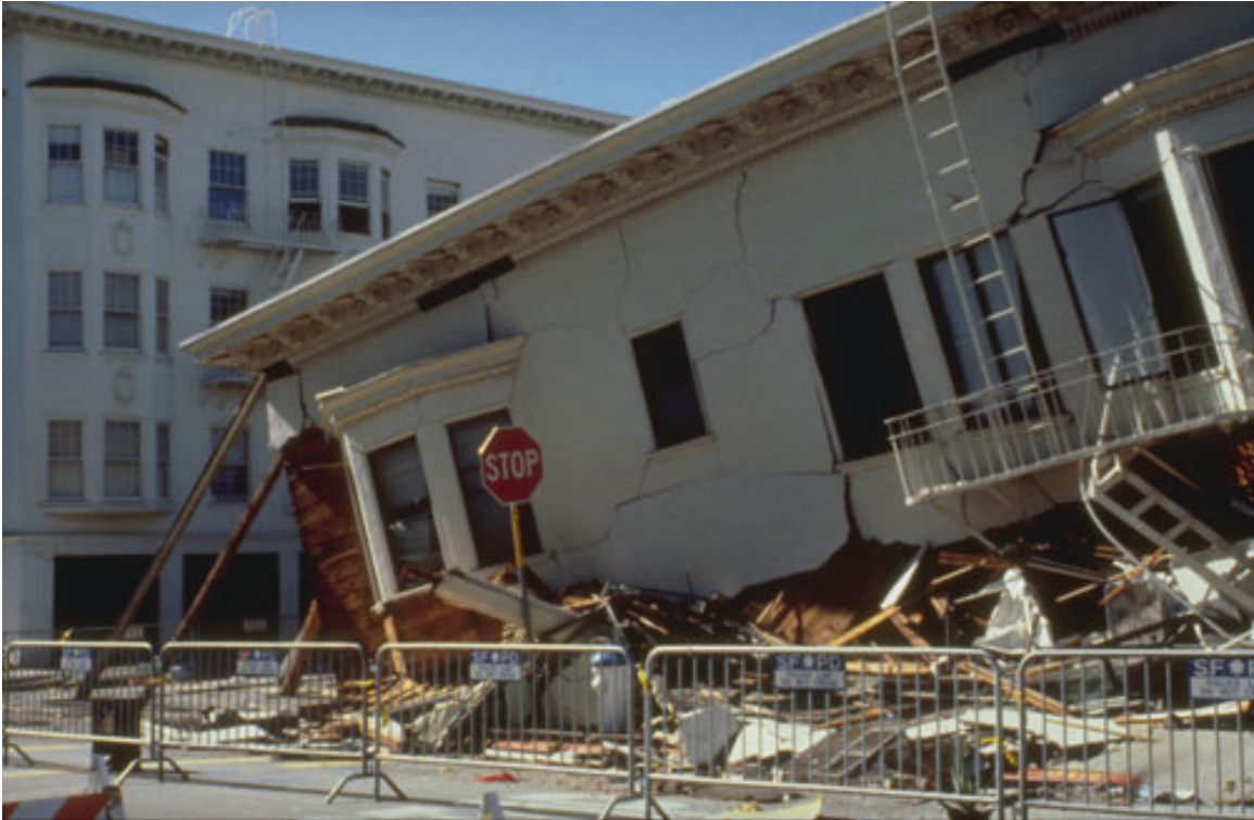
Figure 2. Liquefaction settlement damage caused by Loma Prieta Earthquake, San Francisco, California (1989). Photo downloaded from USGS web site - Liquefaction Hazards Program, Liquefaction Hazard Maps, San Francisco Bay area: http://earthquake.usgs.gov/regional/nca/qmap/
