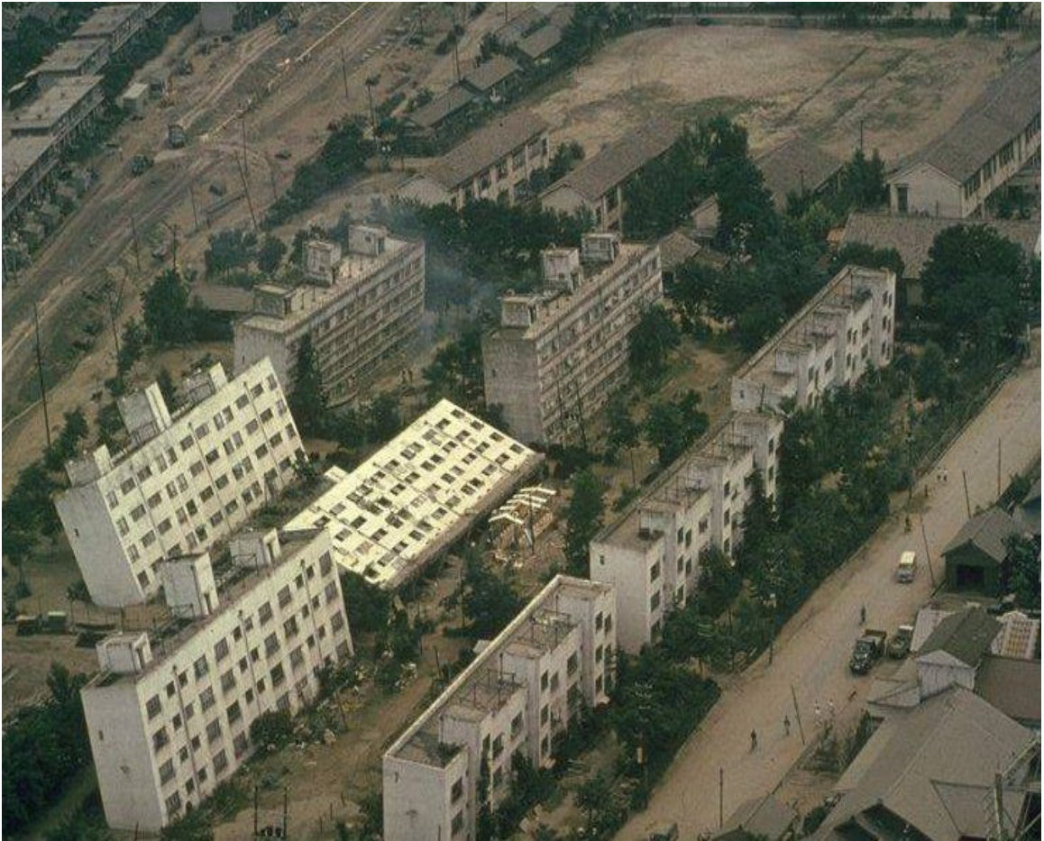
Figure 1. Overturned apartment complex buildings in Niigata, Japan (1964). Photo from the University of Washington Liquefaction web site: http://www.ce.washington.edu/~liquefaction/html/quakes/niigata/niigata.html
