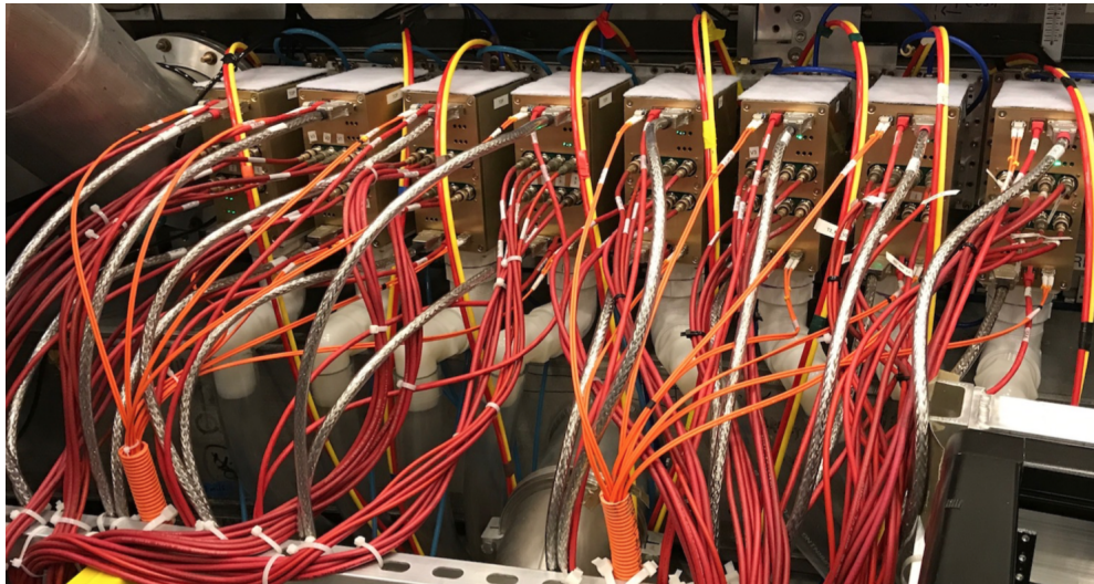
Figure 6.25: A photograph showing an installed tracker station.
