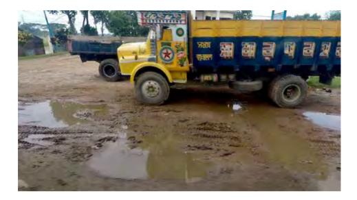
Most roads in Bangladesh experience regular deterioration during the rainy season. Seasonal fluctuations of wetness cause clay soils to shrink and swell, weakening road foundations. Cracks allow water to seep inside, small cracks become large potholes which are worsened by the pummelling of traffic, wind and rain. Through weathering and disintegration brick returns to sediment, creating seasonal cycles of maintenance, fuelling the never-ending demand for brick.
