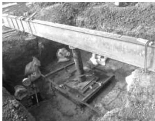
Figure 2.8. Test arrangement for full scale footing test (from Maheshwari et al., 2011).
