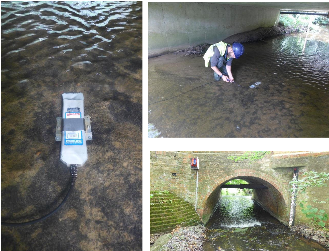
Figure 3.3: Installation of flow monitoring equipment on stream bed in urban culverts.
