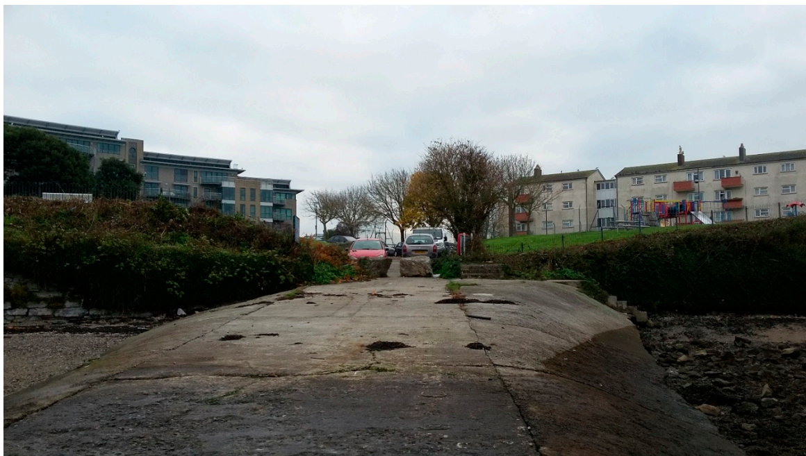
Figure 3. A view from the slipway to the park, with the blocked access, the run-down play area and the social housing in the background to the right. The low cliffs are overgrown with vegetation which blocks views.
