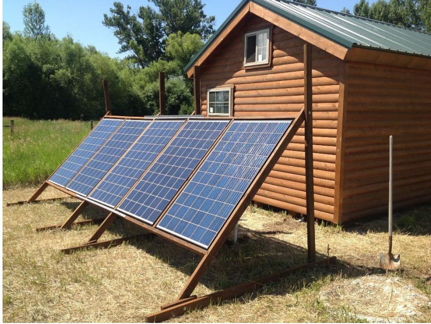
Figure 26 DIY structure designed and installed by Dr. Craig Friedrich (Montana)
