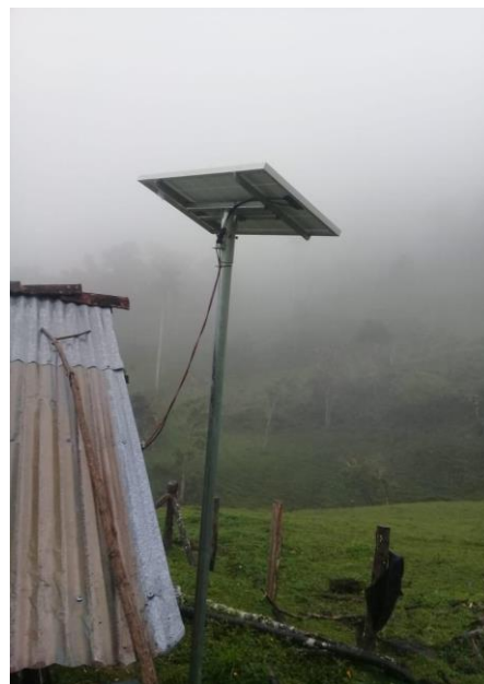
Figure 15 Panel is pole mounted
