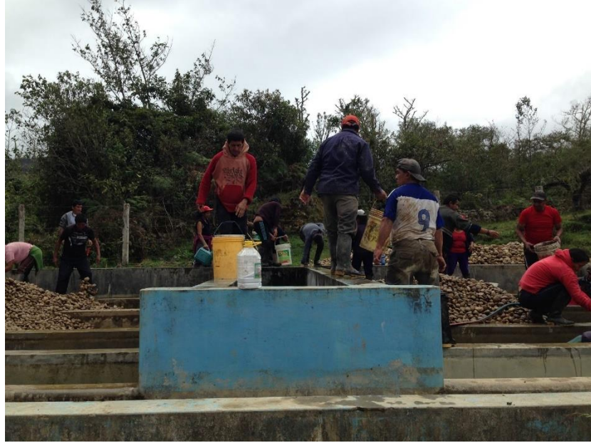
Figure 8 "Minga" for Rehabilitation and Maintenance of Water Filter
