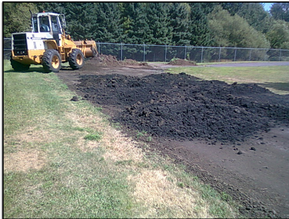
Figure 2-2. Treated sewage solids are termed biosolids. Biosolids can be land applied as a fertilizer or soil amendment.
