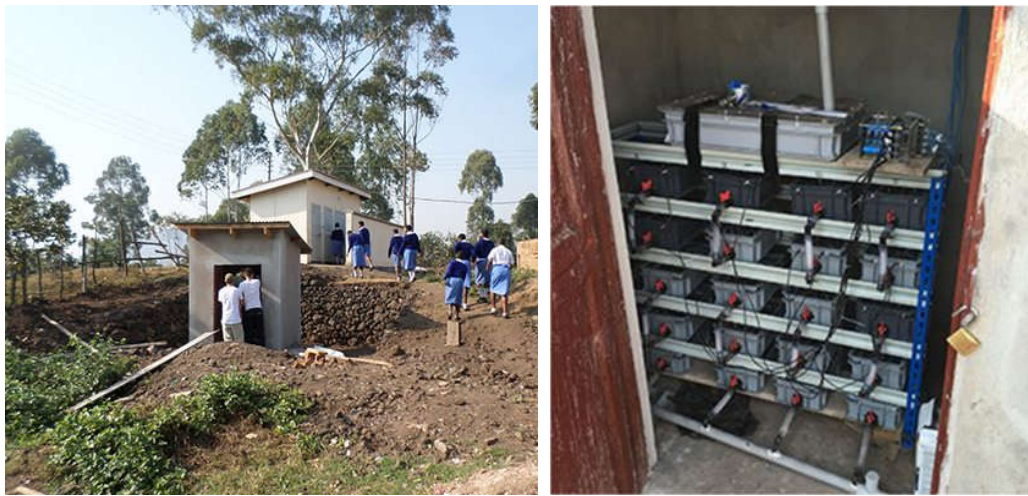
Figure 2. Photographs of Pee Power installation site (left) and system (right). In the left photo, building block located on the lower ground is where the Pee Power system was installed. The building on upper ground is an existing toilet block of the Seseme Girls' Secondary School.
