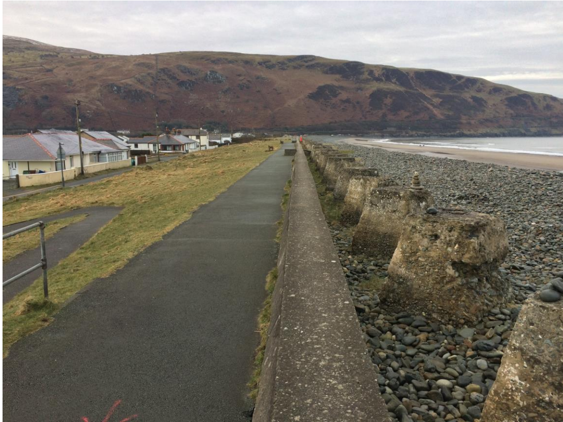
Figure 3: Sea defences at Fairbourne (Source: Author). Policies based on the SMP2 propose to maintain this infrastructure for about 40 years after which point the coast will be realigned.
