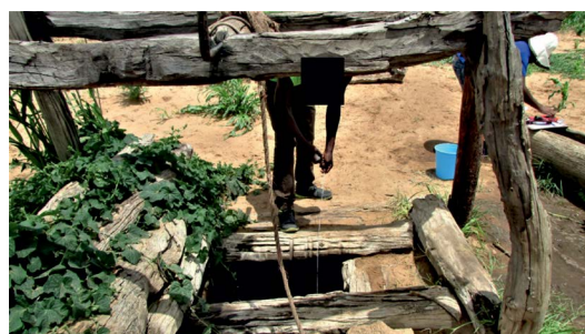
Fig. 3. A picture of type 3 deep hand-dug wells found in Ohangwena and Omusati regions of the CEB in which animals cannot walk into the water.
