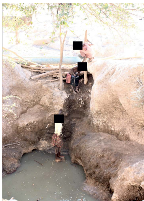
Fig. 2. A picture of type 2 shallow hand-dug wells found in Ohangwena and Omusati regions of the CEB in which animals cannot walk into the water.
