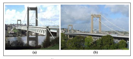
**Figure 2.** Tamar suspension bridge (a) before (1978)<sup>36</sup> and (b) after (2018) its reconstruction in the late 1990s. Note the larger deck and stay cables added in 2001.
