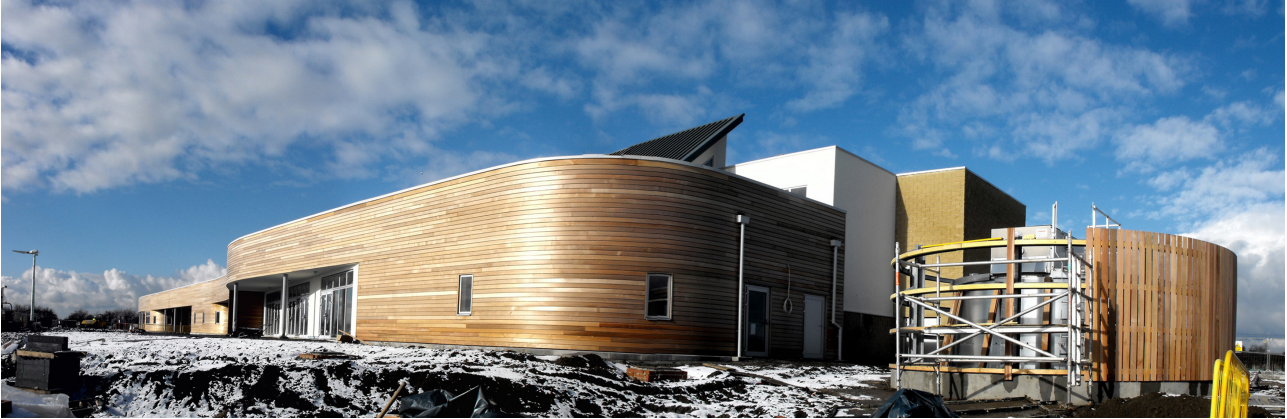
fig 3. Construction photograph of the energy centre, John Ferneley College.
