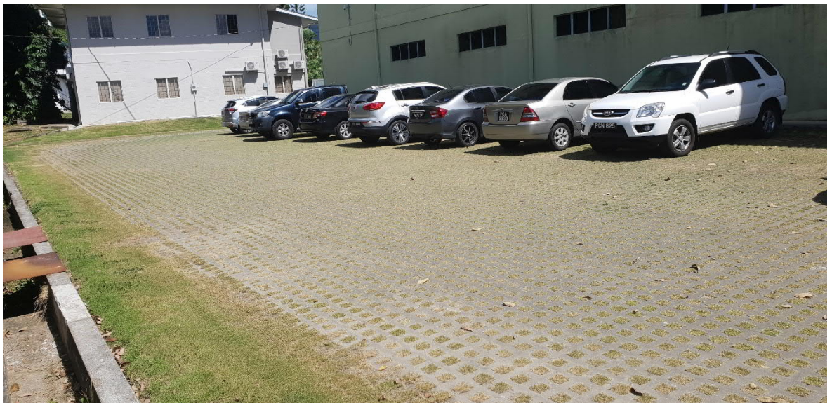
Figure 2-12 Grass-infilled concrete grid pavers at the University of the West Indies, St. Augustine Campus, Trinidad, W.I.
