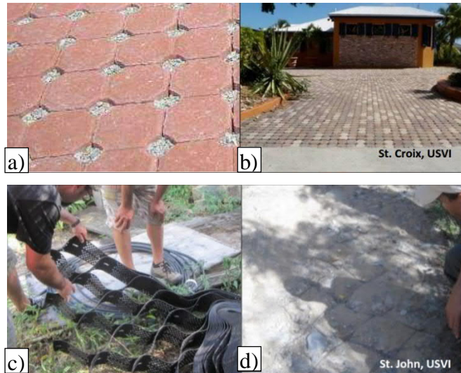
Figure 2-11 PPS in Caribbean islands (a) and (b) PICP with apertures at St. Croix, (c) and (d) PG in St. John, USVI
