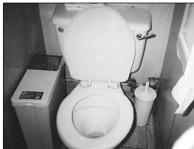
Fig. 4. Lack of coordinated decision making results in cluttered cubicles with bins too close to the toilet seat
