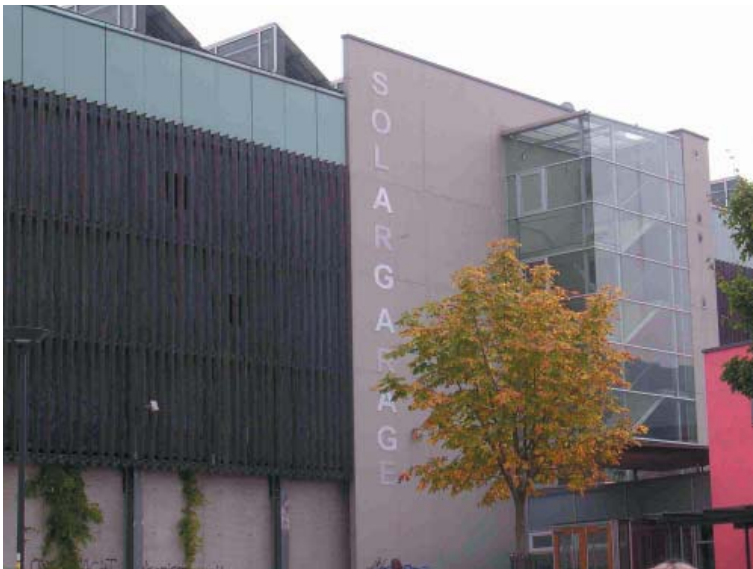
Large garage at edge of Vauban for residents parking
