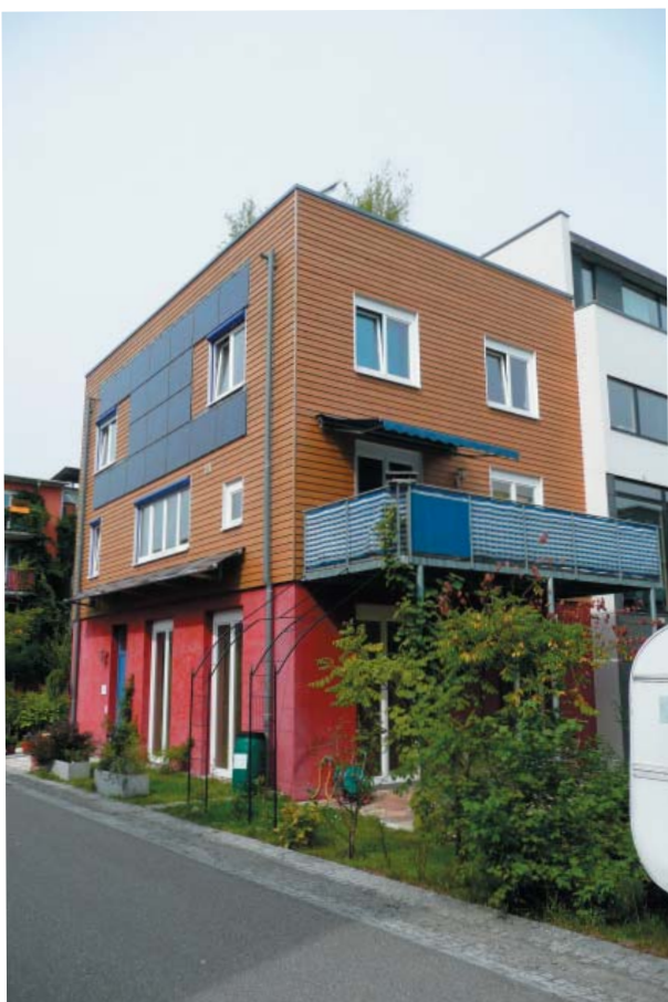
Solar photovoltaics on house in Vauban
