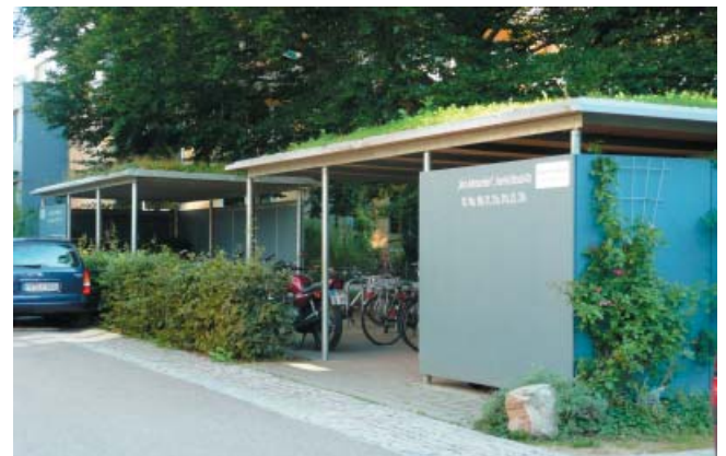
Well designed communal bike sheds for residents
